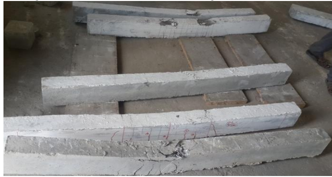
Figure 8. Reinforced concrete beams after testing. Source: Self-Elaboration.
