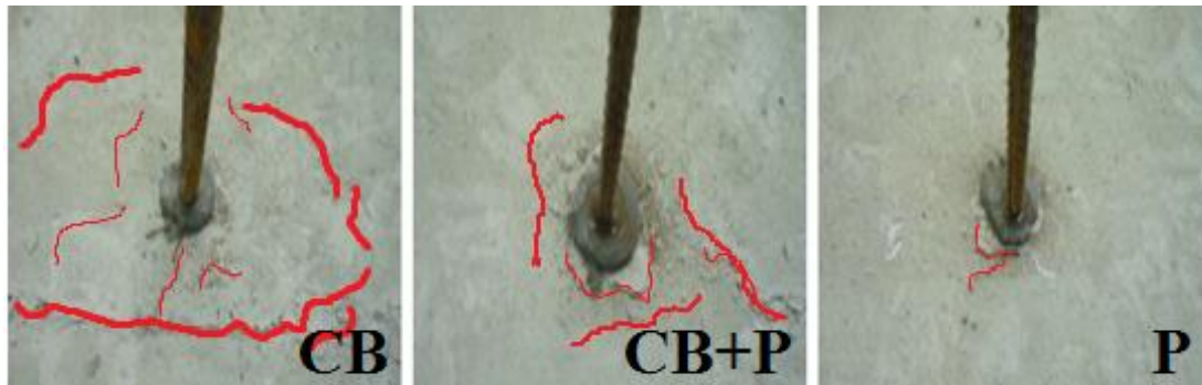
Figure 6. Image for the test samples (CB: concrete breakout, P: pull-out).
