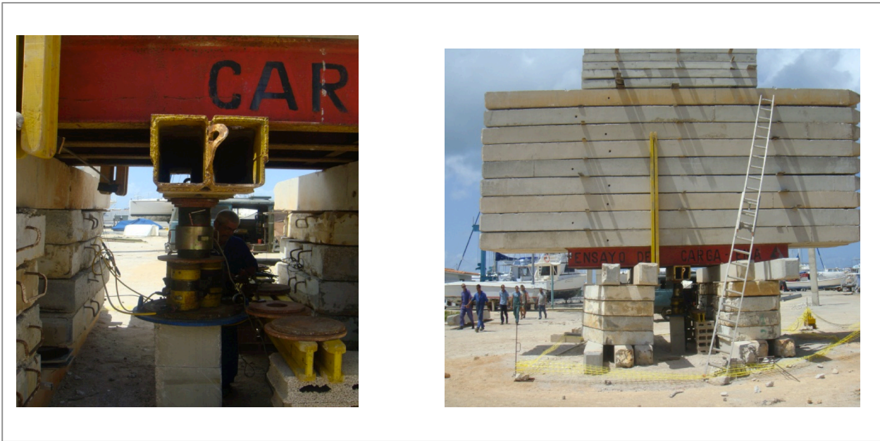
Figure 3. Photos of conducting load tests
