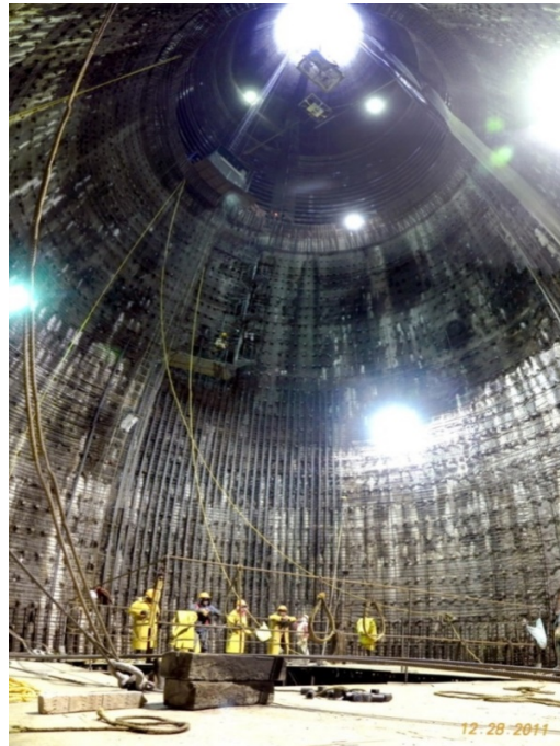
Figure 7. Assembly of the grids in the heights
