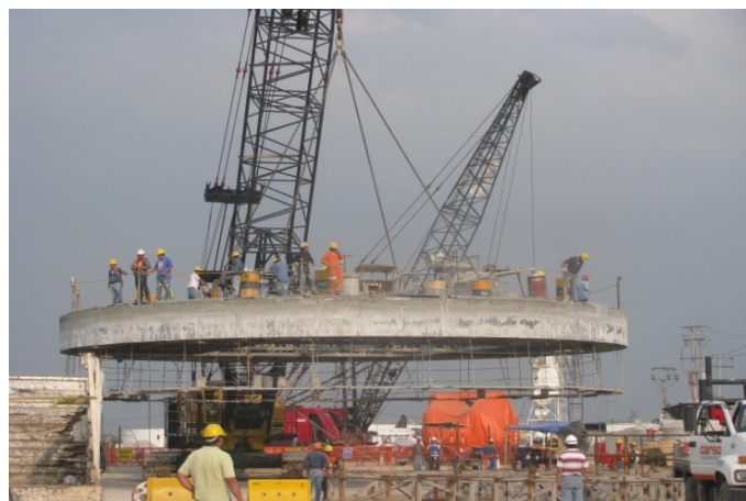
Figure 8. Assembly of the sliding formwork
