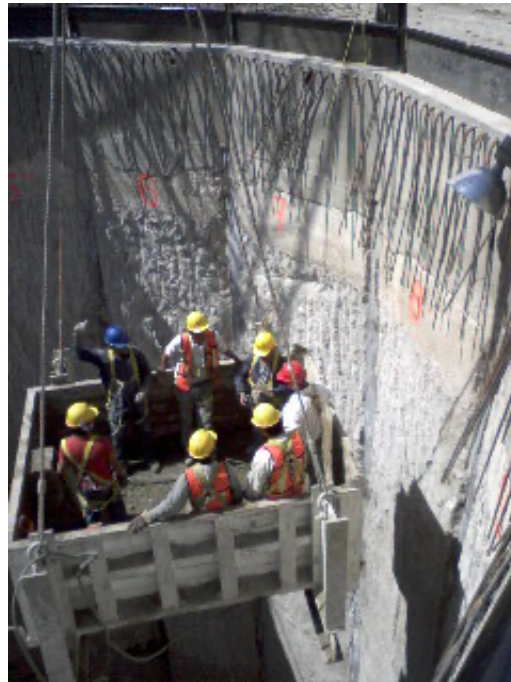
Figure 4. Workers' descent in an improvised bucket
