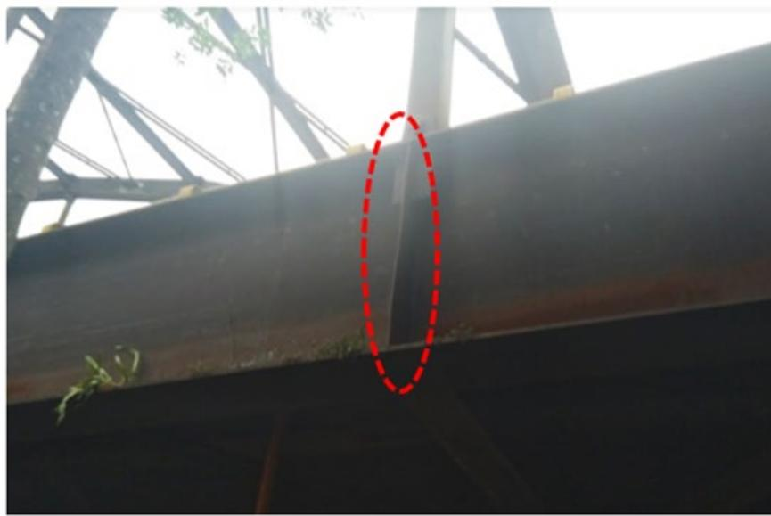
**Figure 7.** Local buckling of a web stiffener just at the point of a hanger's connection area for the Unete steel arch bridge
