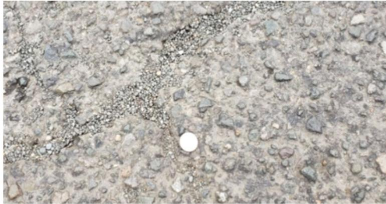
**Figure 13.** Surface damage for CDD=154.593 °C-days
