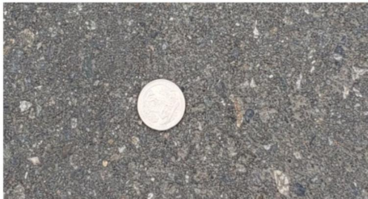
**Figure 9.** Surface damage for CDD=42.079 °C-days
