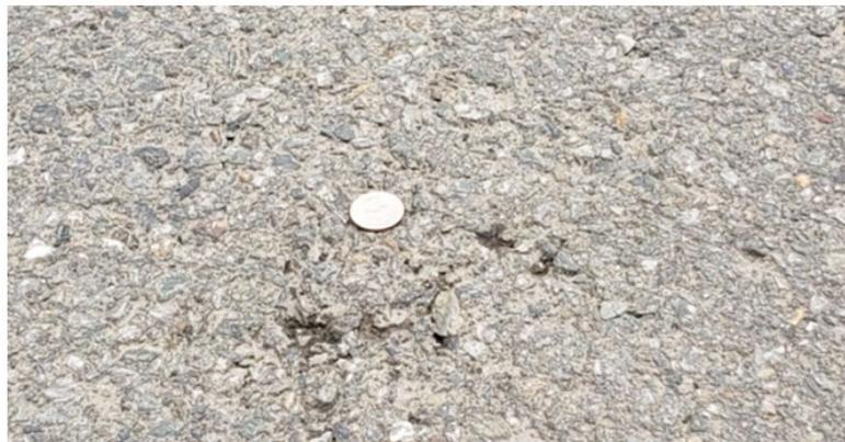
*Figure 12. Surface damage for CDD=80.498 °C-days*
