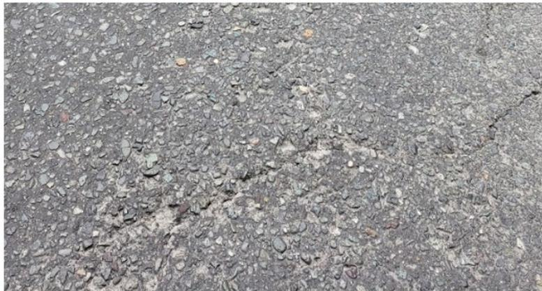
*Figura 11. Surface damage for CDD=74.112 °C-days*
