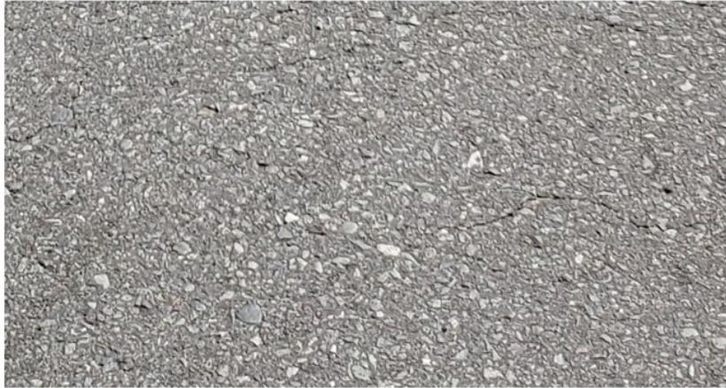
*Figura 10. Surface damage for CDD=51.482 °C-days*
